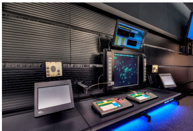
Room to relocate or add new equipment
